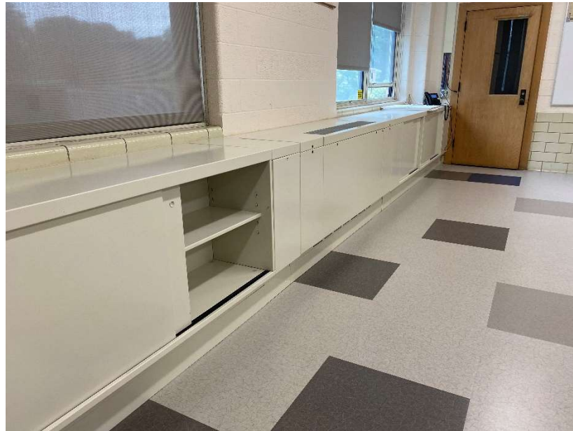
New mechanical (unit ventilators)
