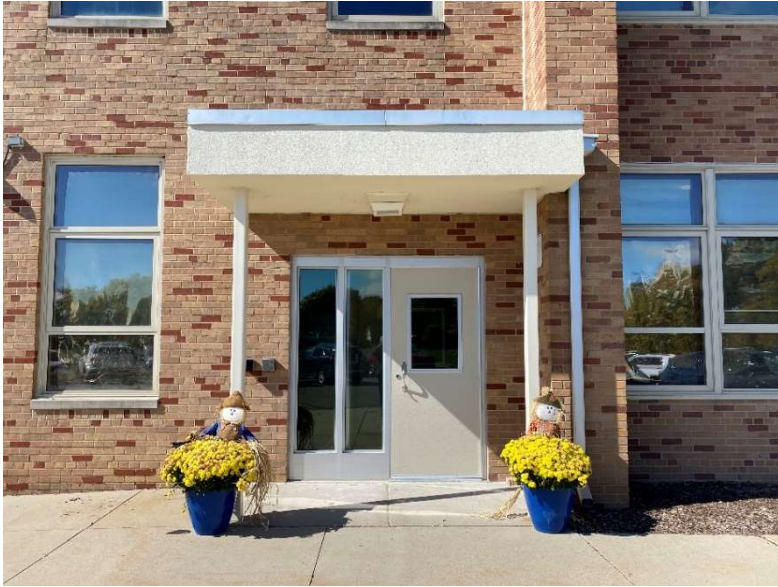
New secured vestibule
