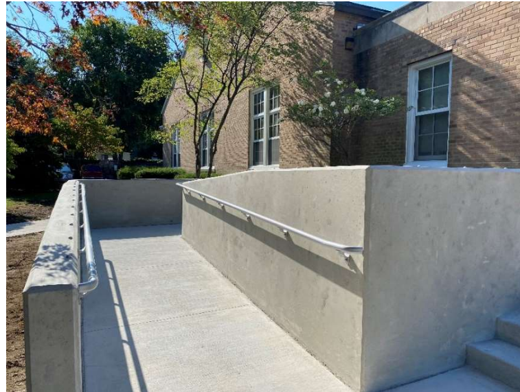
New ADA compliant ramp
