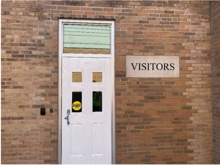
New secured vestibule
