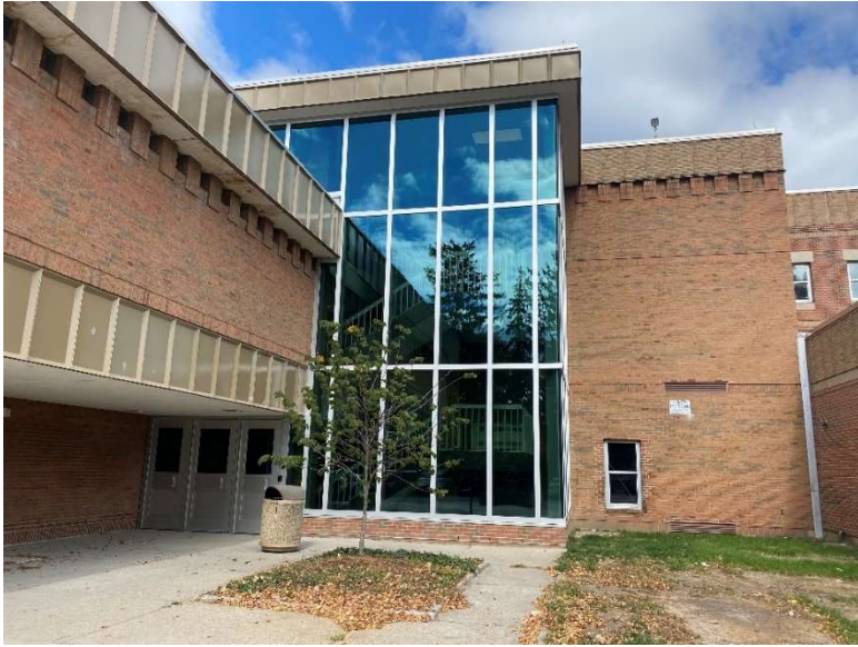
New stairwell windows
