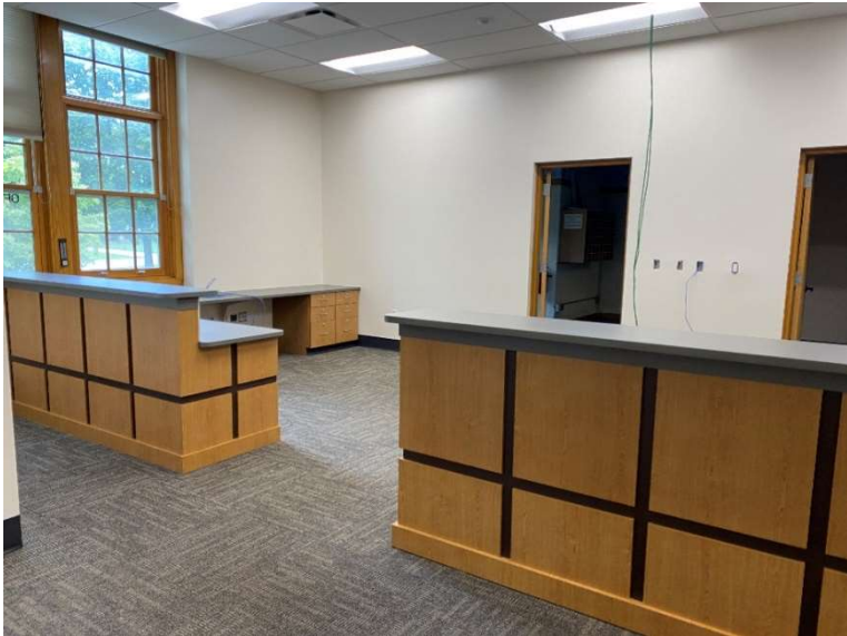
New secured vestibule
