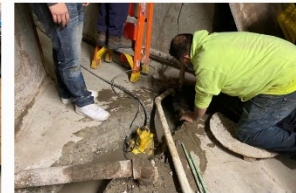
GP South Tunnel Repairs
