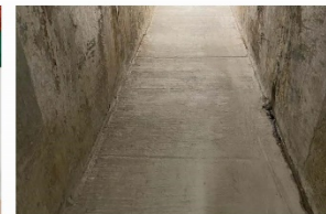
GP South Tunnel Repairs
