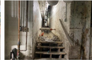
GP South Tunnel Repairs
