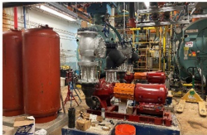
GP South Mechanical Equipment Install
