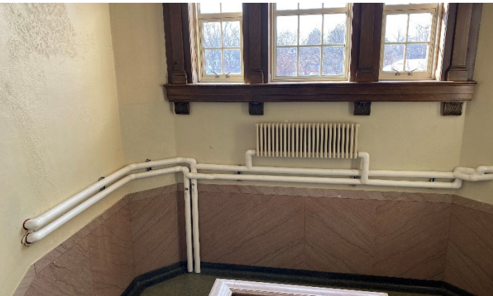
Stairwell Hydronic Pipe
