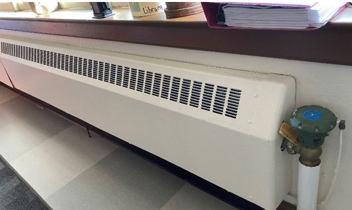
Steam Fin Tube Exterior Wall Heating
