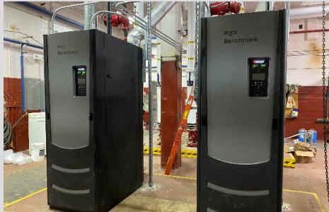
Condensing Boilers
