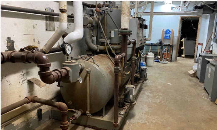
Mechanical Room Steam Condensate Tank
