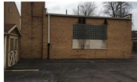
Water Staining on Brick
