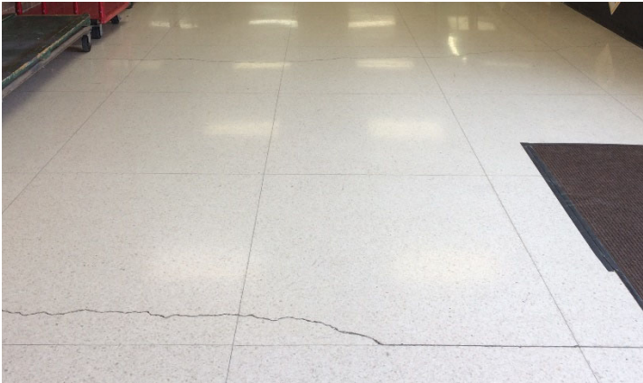
Floor Cracks
