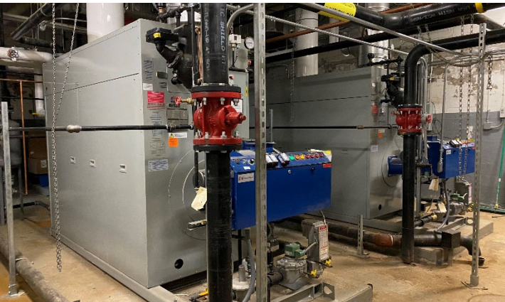
New Mechanical Room Steam Boiler
