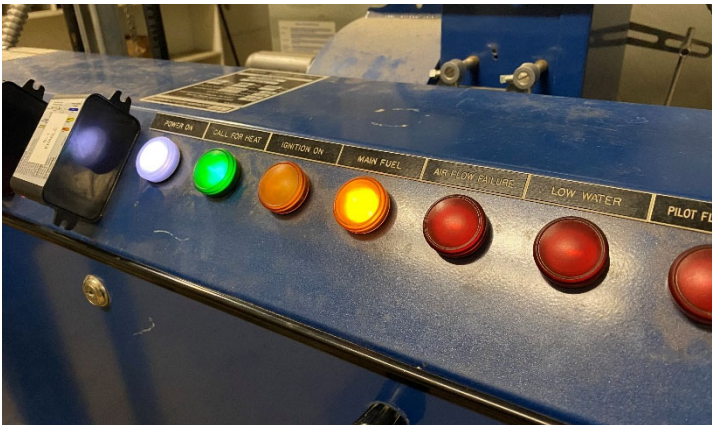
Steam Boiler Controls
