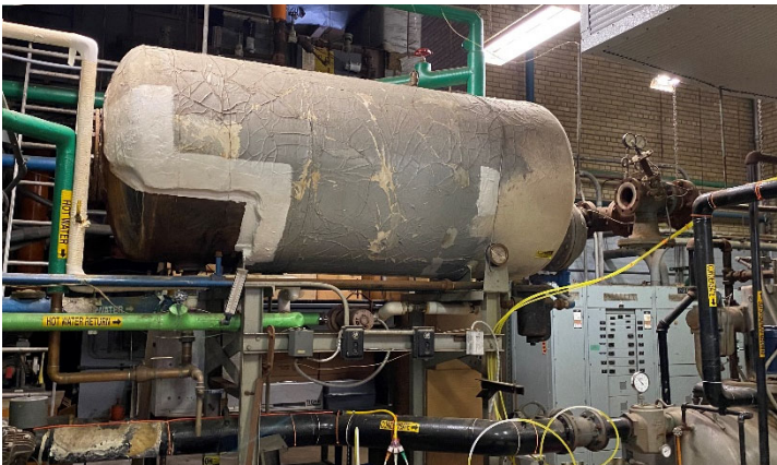
Steam Condensate Tank
