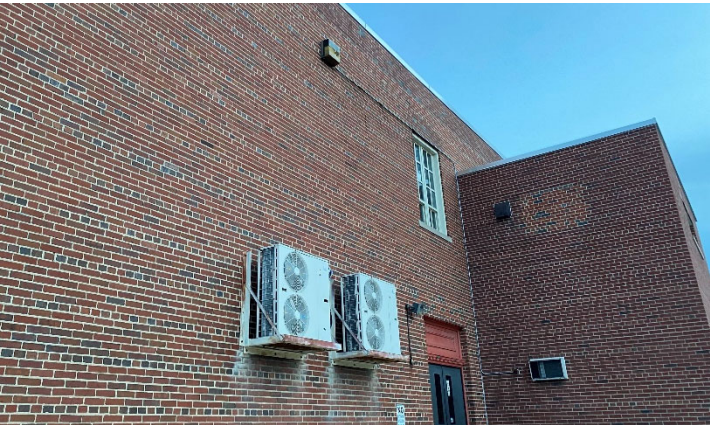
A/C Condensing Units
