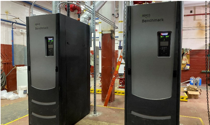
Condensing Boilers
