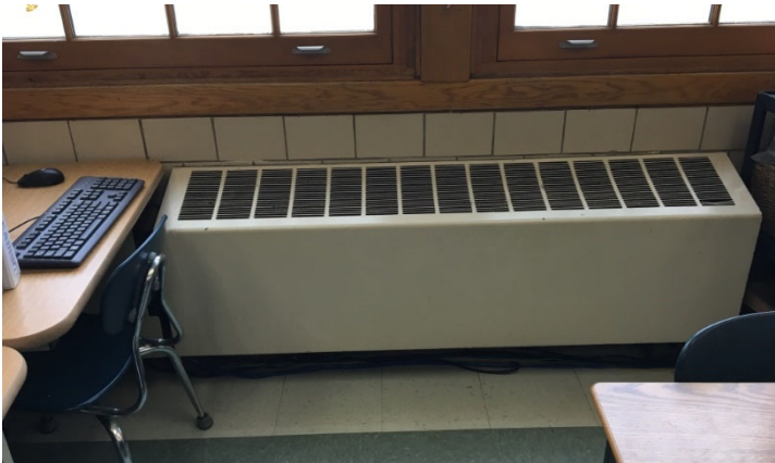
Exterior Wall Unit Heater
