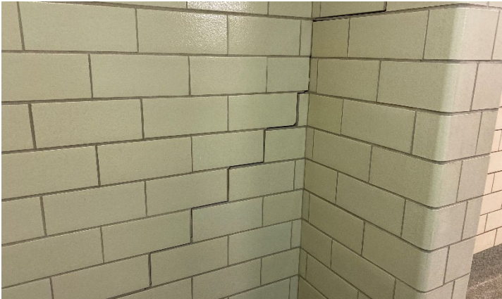
Locker Room Wall Tile Crack
