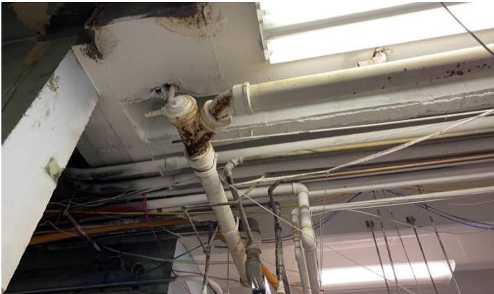
Cast Iron Drain Pipes
