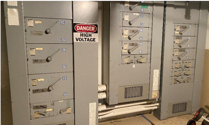
Electrical Switch Gear
