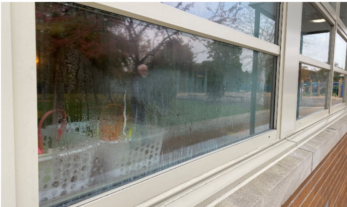
Broken Window Seal
