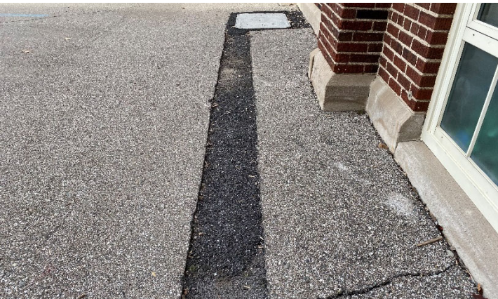
Building Fiber Install Patch
