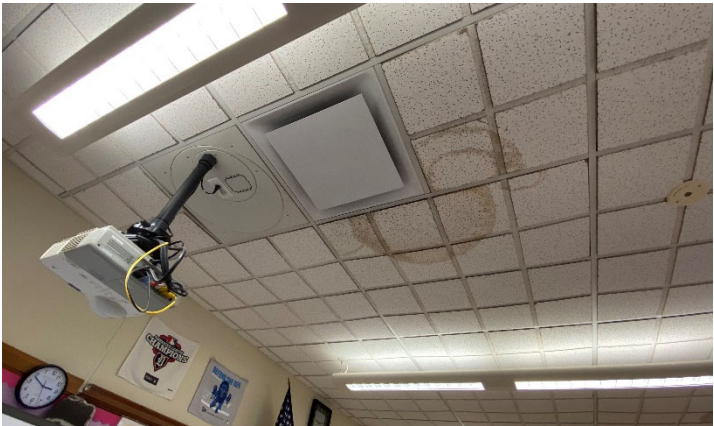
Science Lab Ceiling Leaks
