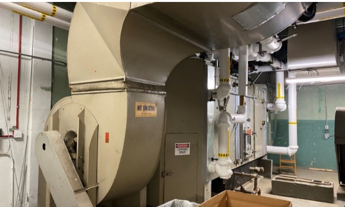
Air Handling Unit Duct Work
