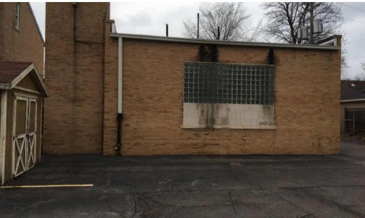
Water Staining on Brick
