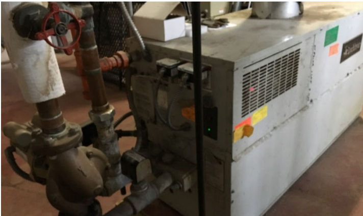
Domestic Hot Water Boiler
