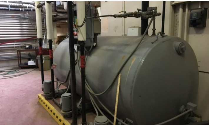
Steam Condensate Tank
