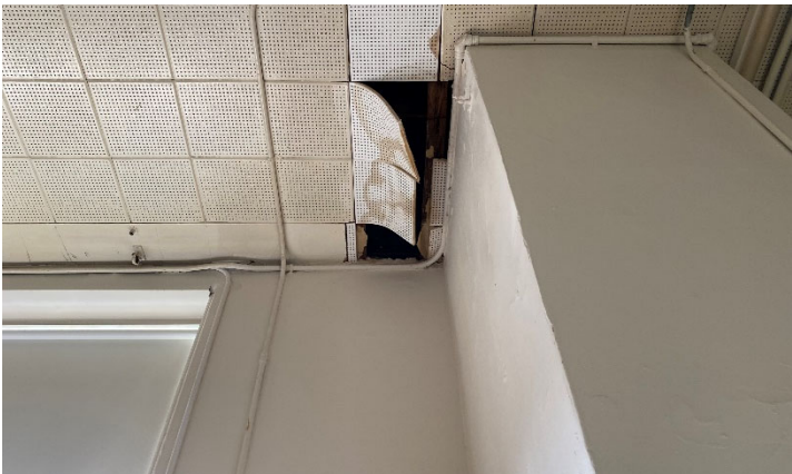
Kitchen Ceiling Damage
