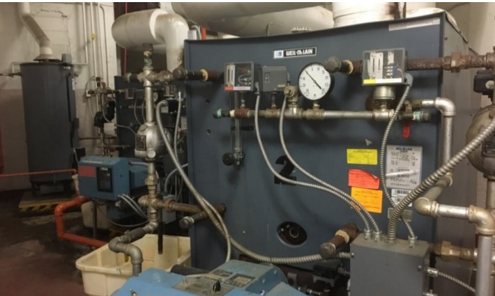
Steam Boilers (will be changed to hydronic in 2022)
