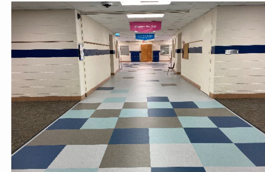
Ferry Corridor Flooring
