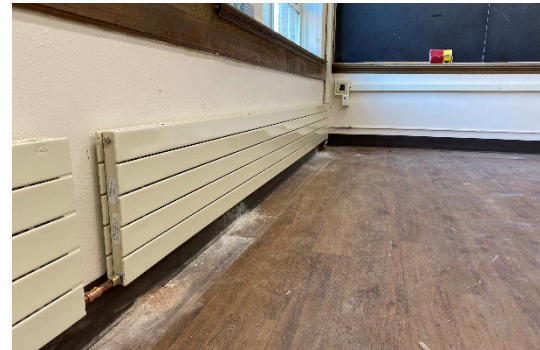
GP South Hydronic Radiant Panel Install
