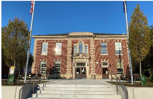
GP South Fisher Plaza Main Entry
