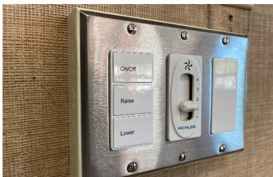
GP South Classroom Controls
