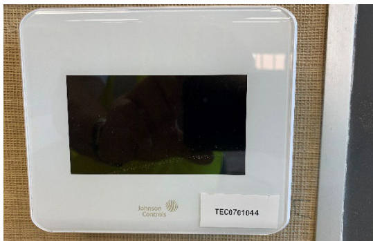
GP South Temperature Controls
