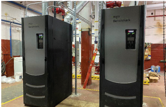
New Hot Water Condensing Boilers
