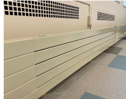
Hydronic Heating System - Ma
